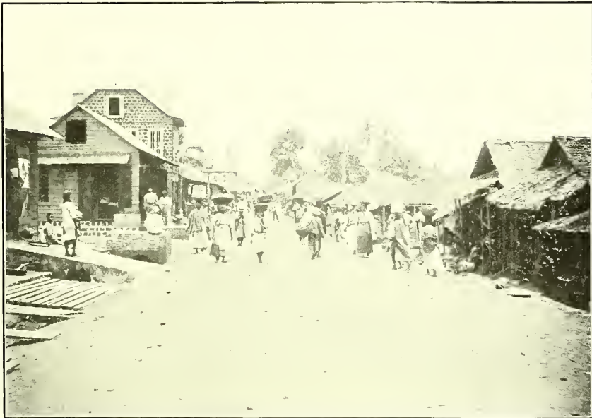
A STREET IN FREETOWN, SHOWING DRAIN AT SIDE AND NUMEROUS GANGWAYS OVER IT. HOUSES ON RIGHT SIDE ARE LOWER THAN STREET LEVEL.
