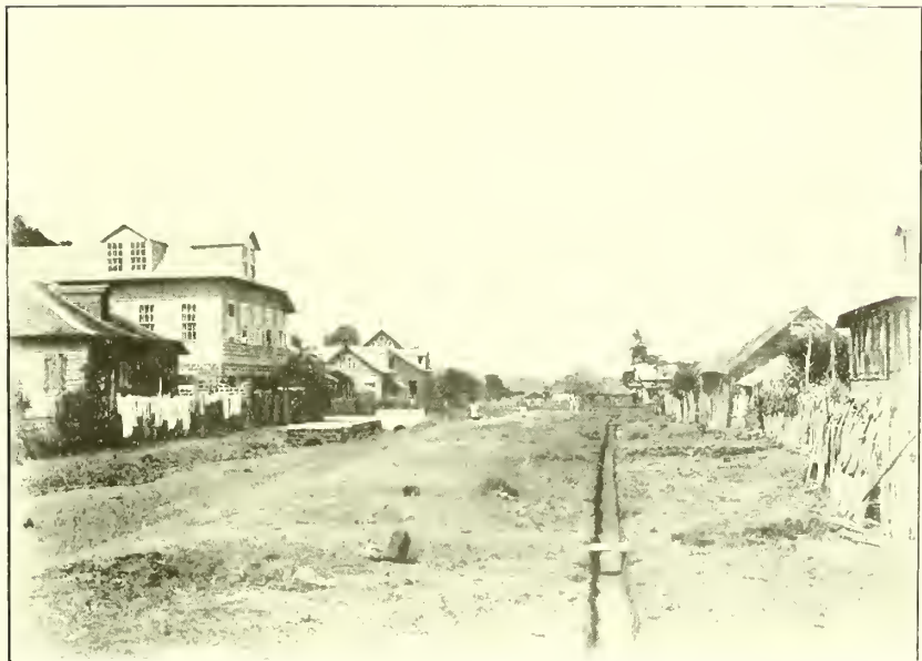
A STREET IN GRASSFIELDS, FREETOWN, SHOWING DRAIN CUT OUT OF THE ROCK AND ROAD MADE UP, SO ABOLISHING STREET POOLS
